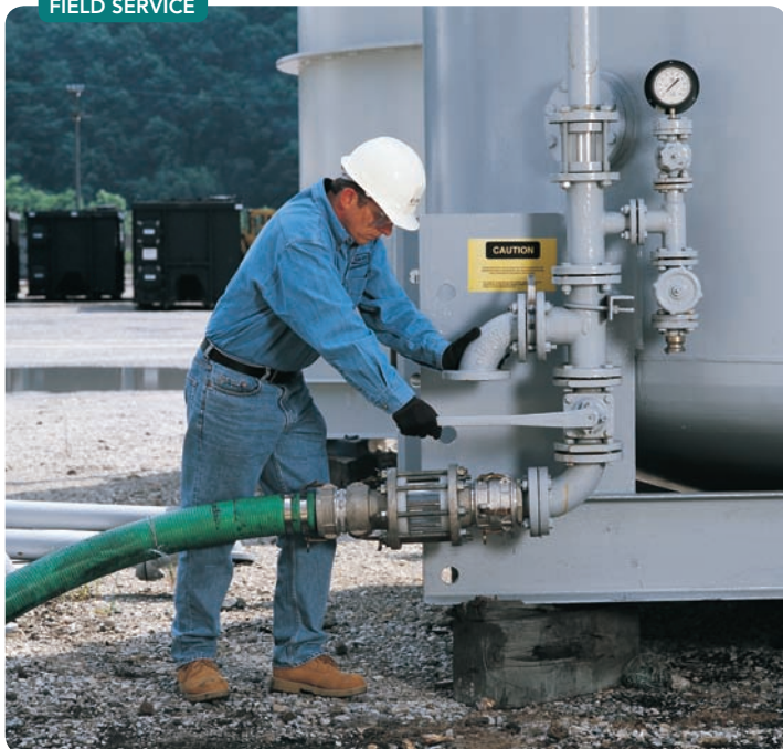
Figure 1. Vendor usually handles the installation of fresh activated carbon.
